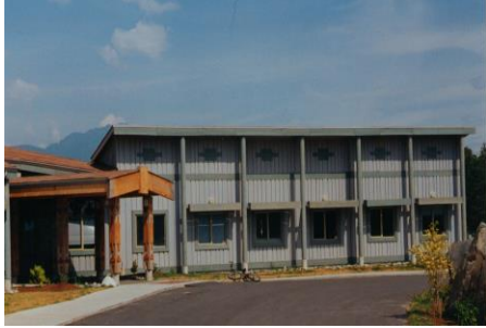
figure 50 seabird island administration & recreation building (© patrick r stewart architect 1996) reprinted with permission
