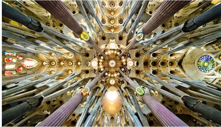
figure 32 the nave in the sagrada familia looking up at its hyperboloid vault
